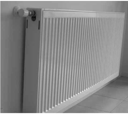
Figure 2: Hydronic heating system
