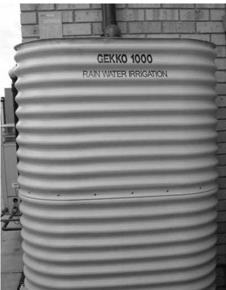
Figure 3: Rain water tank (1000 litres) for roof runoff collection
