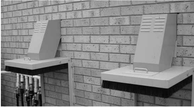
Figure 4: Separate collection chutes for recyclables and organic waste from kitchen.
