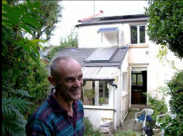
Large south facing areas of PV and solar thermal
