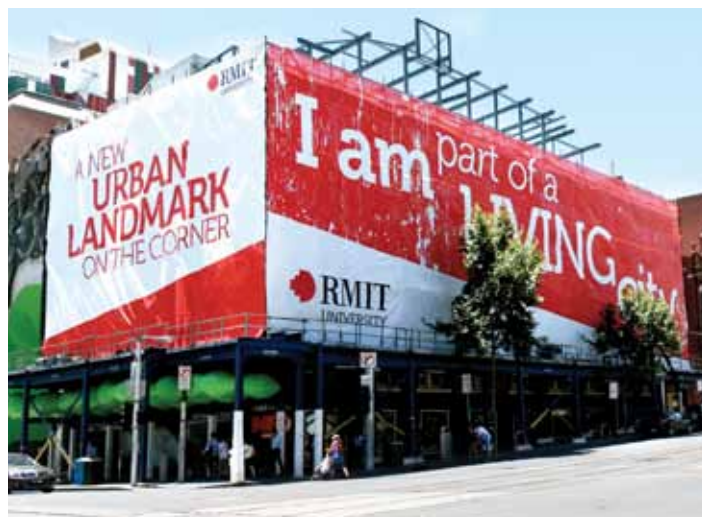
Building 22 on the corner of La Trobe and Swanston Streets. Property Services gets creative with hoarding to promote the RMIT brand.
