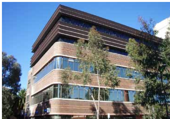
Building 9 has been extended by two levels.
