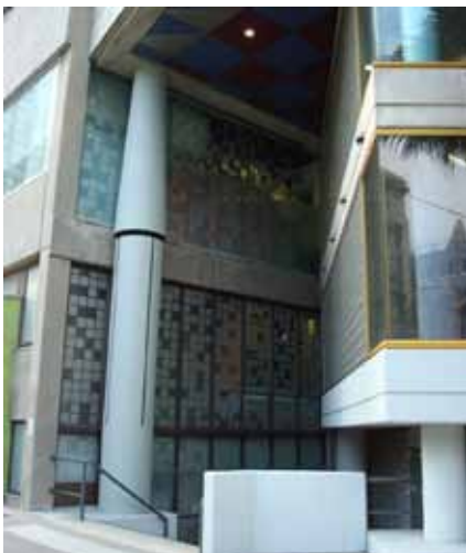
Building 10 windows on Swanston Street have been enhanced with the RMIT University logo and a pixel motif in a semi-opaque decal film.
