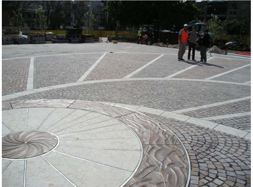
Piazza Italia, Carlton: Grey and red (rosso) porphyry cobblestones in traditional overlapping arcs, with the central sundial in bronze, stainless steel and bands of white verdello stone. Designer: Andreas Tomaselli, 2005
